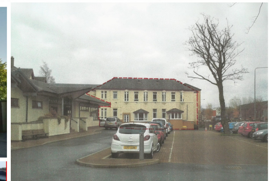
Katrine House : Existing Building to be Demolished ( Building marked with broken red line)
